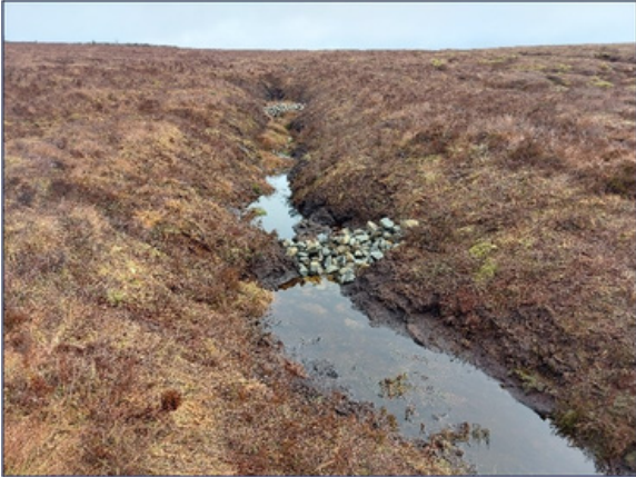
Photo 5: Installed stone dam
