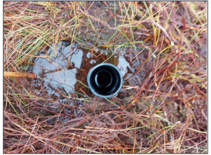
Photo 10: Dipwell installed for monitoring water table levels.
