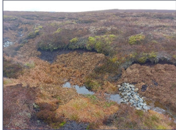
Photo 6: Installed stone dam with heather brash spread around the area
