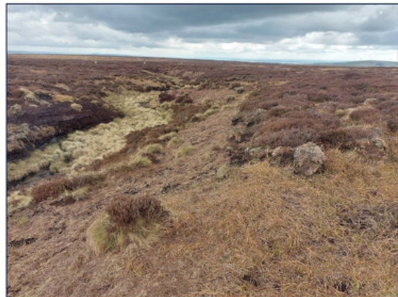
Photo 8: Heather brash and seed spread on reprofiled gully edge.
