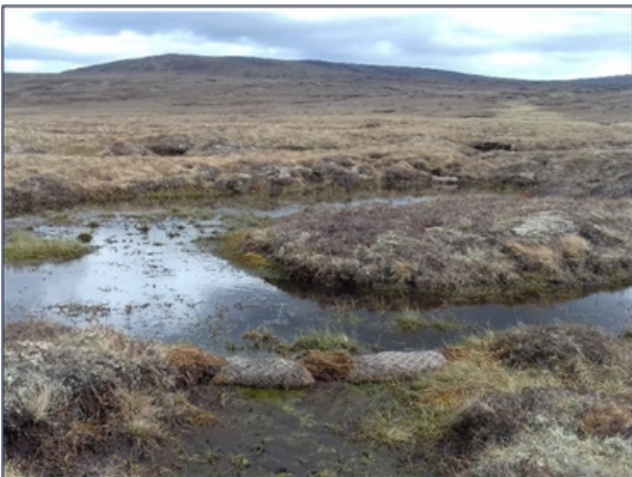
Photo 7: Coir dams dividing large area of bare peat into smaller units.
